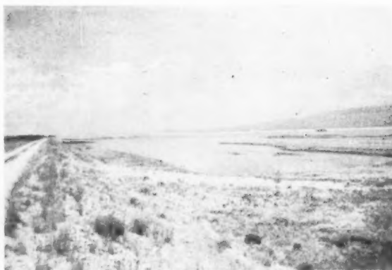
SETTLING POND where soluble iron in Silver Bow Creek water is precipitated out by lime in mill tailing water.
